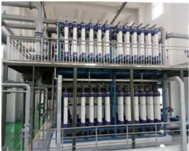
60000T/D Reservoir Upgrading in Qingdao
