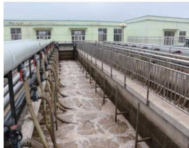
40000T/D Wastewater Plant Renovation in Lingang
