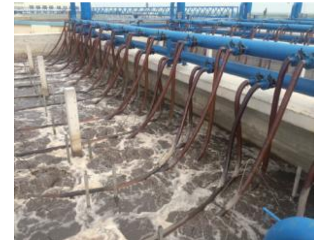
25000T/D Shengjie Sewage Plant Renovation
