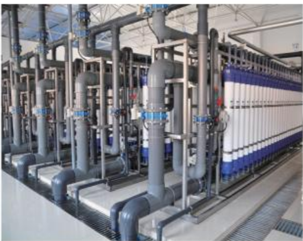
10000T/D Reservoir Upgrading in Dongbei
