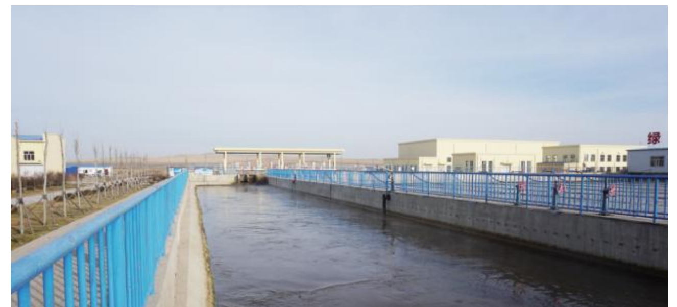
30000T/D Sewage Plant Renovation in Inner Mongolia
