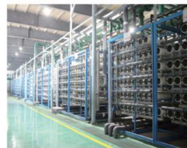
17280T/D Steel Company project in Tianjin
