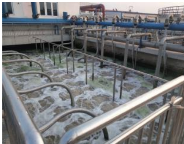
40000T/D Sewage Plant Renovation in Hebei
