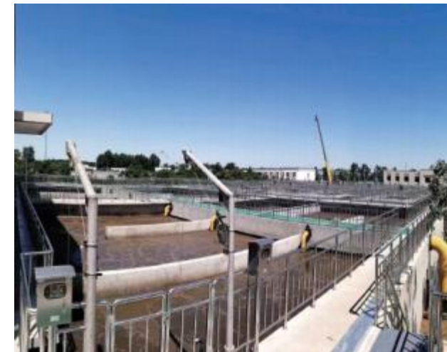
50000T/D Sewage Plant Renovation in Sanhe
