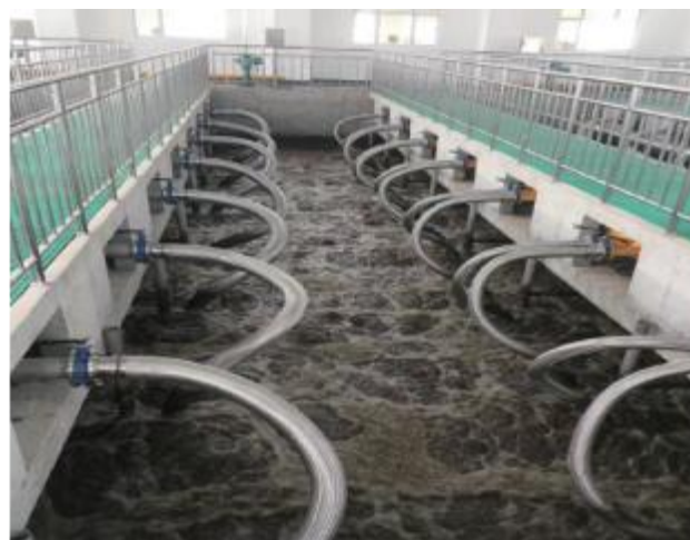
25000T/D Sewage Plant Renovation in Cangzhou
